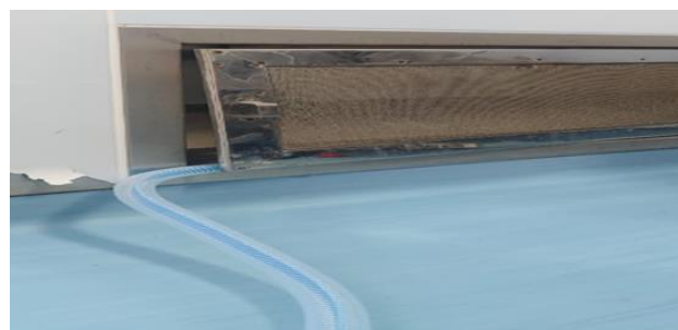
Fig-1: Release the oxygen cylinder pressure into the air conditioning outlet through a long circuit
